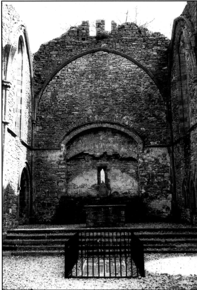
The Abbey Church chancel with the tomb of Fr Ignatius OSB in the foreground. The altar dedicated to the late Fr John Windle of Welsh Newton is at the presbytery end. The towering East wall is now badly cracked and dangerously unstable.
